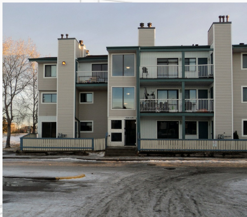
Exterior of building with large shared use parking
